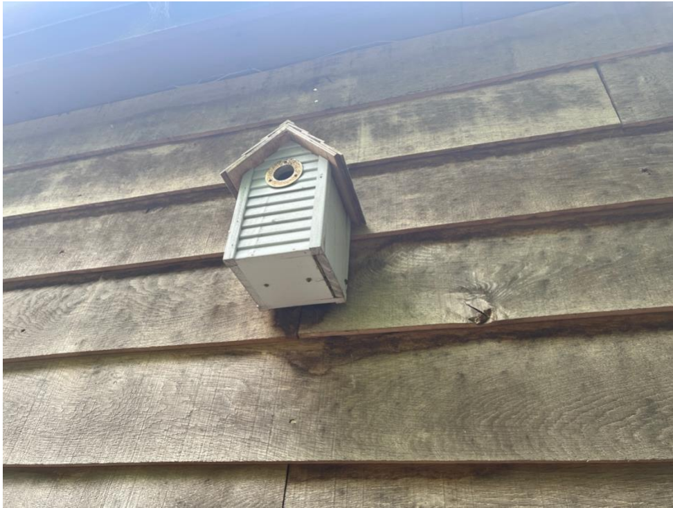
Figure 4: Example of bird box on site
