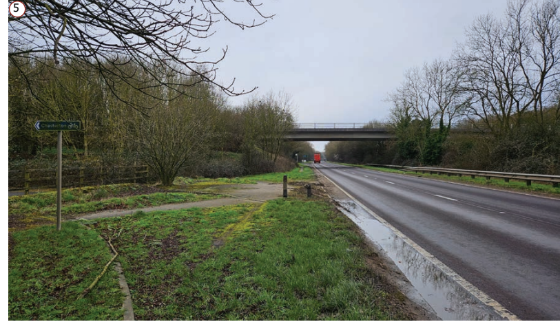
FIG 18- VIEW OF BLOCKED OFF SLIP ROAD ENTRANCE FROM A41
