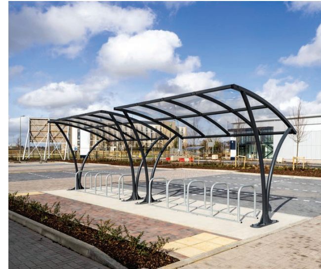
FIG 52- CYCLE SHELTERS AT UNIT1, CATALYST DEVELOPMENT
