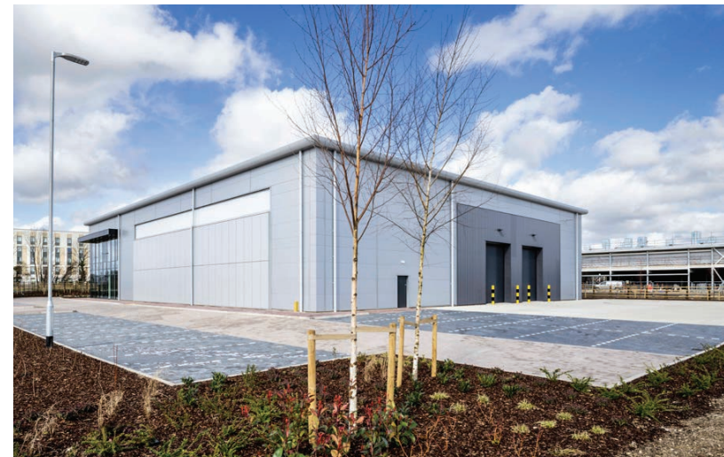
FIG 48- PRECEDENT IMAGES OF MATERIALS AND ARCHITECTURAL FEATURES, SUCH AS DOUBLE HEIGHT CURTAIN WALLING AND THE BLACK FEATURE CANOPY, USED ON THE FACADES OF NEIGHBOURING CATALYST DEVELOPMENT
