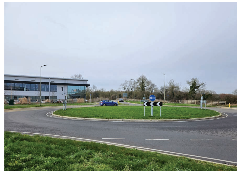
FIG 5- PHOTOGRAPH OF WENDLEBURY RD ROUNDABOUT, CATALYST PHASE 1 TO THE LEFT AND THE VACANT SITE TO THE RIGHT
