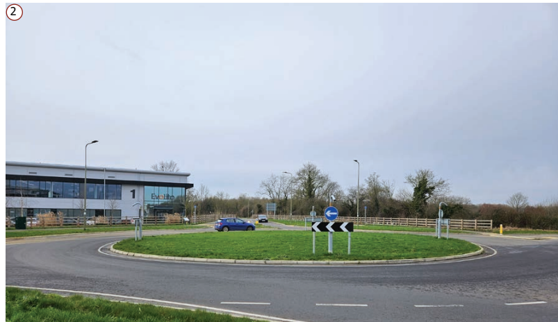
FIG 13- VIEW OF NEWLY IMPLEMENTED ROUNDABOUT AT INTERSECTION OF CHARLES SHOULER WAY AND WENDELBURY RD
