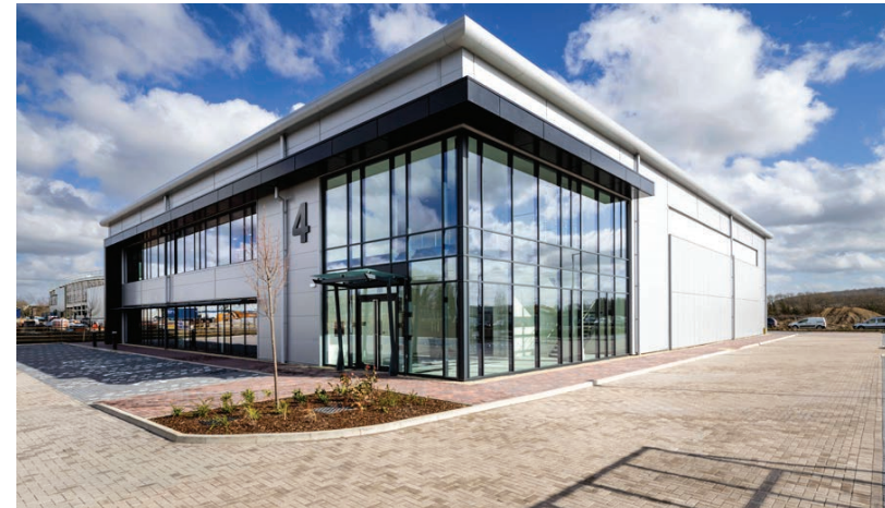
FIG 25- CATALYST - UNIT 4 ENTRANCE, WENDLEBURY RD
