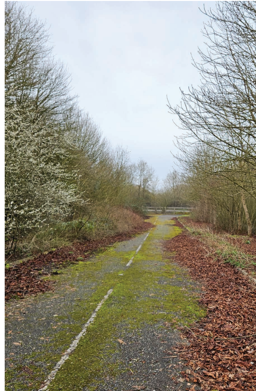
FIG 1- PHOTOGRAPH OF UNUSED/ BLOCKED SLIP-ROAD AT SITE, ACCESS FROM A41
