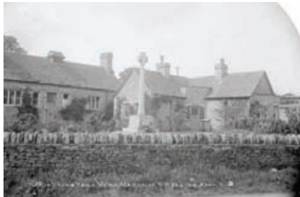
Figure 25 Historic walling in front of the Kirtlington war memorial and reading room, 1920-30. Source: Kirtlington Conservation Area Appraisal.
