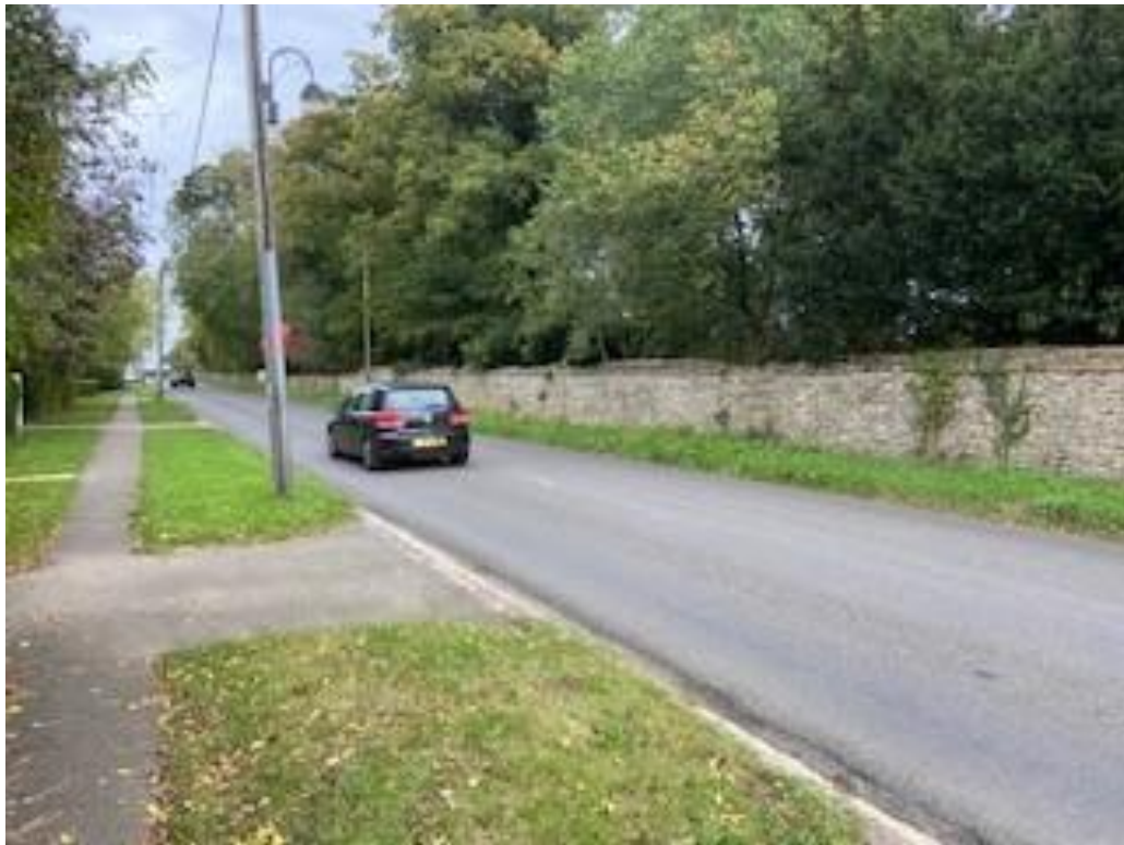
Figure 16 – View north along frontage of site in Heyford Road.
