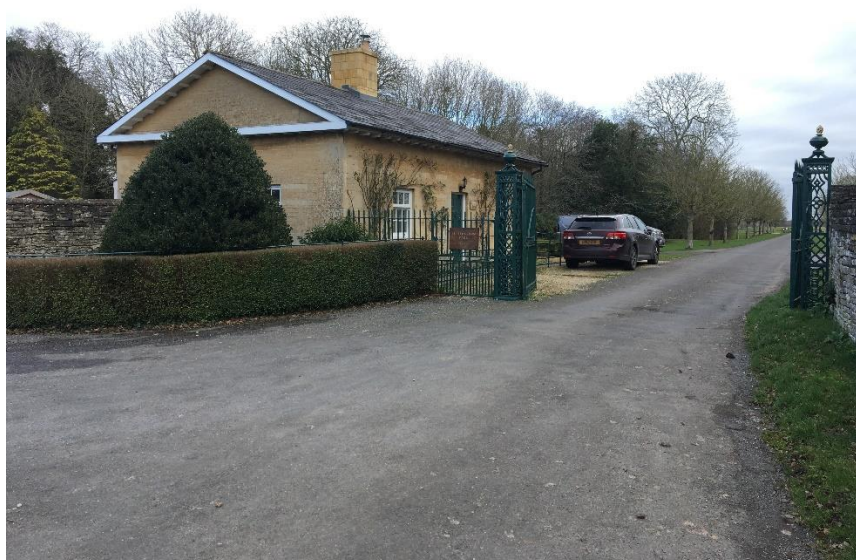
Figure 34 – North Lodge, as viewed from Heyford Road.
