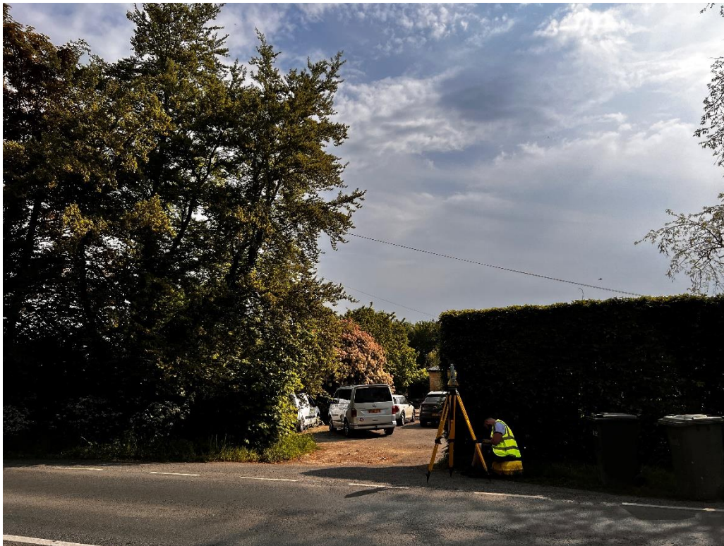
P1 – View of the existing vehicular access to Stable Lodge and The Rectory from Oxford Road
