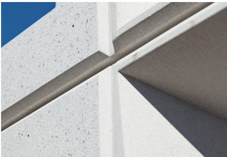
Slab Edge: pre-cast white concrete - acid etched
