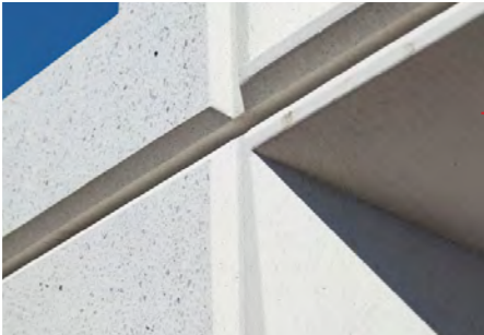
Slab Edge: pre-cast white concrete - acid etched
