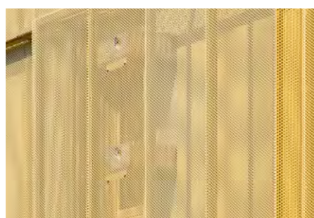
Shading Elements: Perforated anodized aluminum, brass colour, brushed
