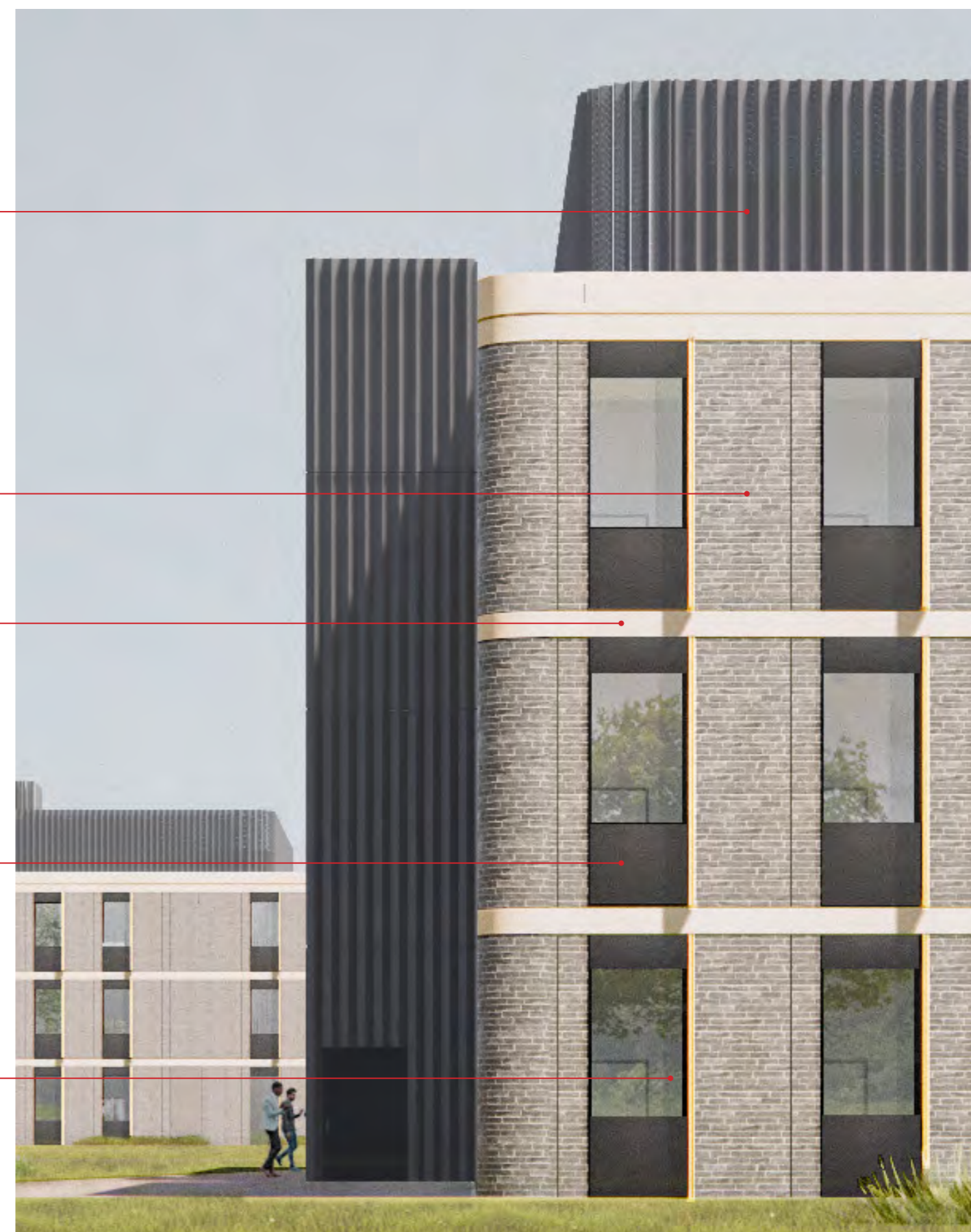
Shading Elements: Perforated anodized aluminum, brass colour, brushed
