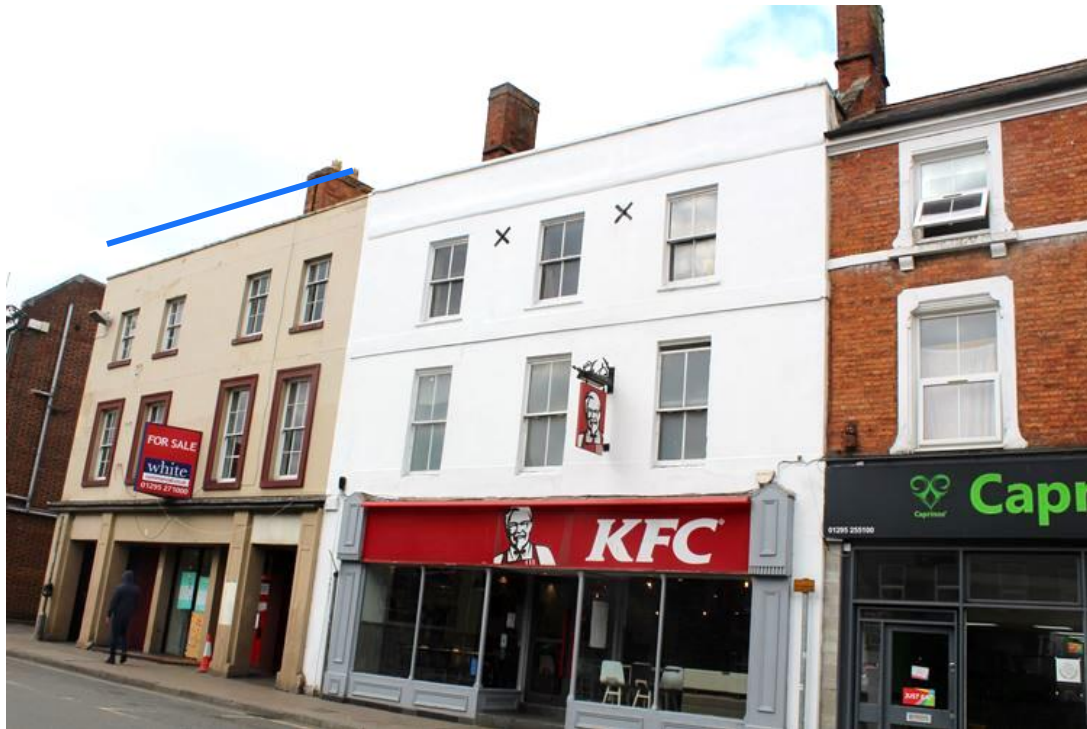
Figure 27: Post Office Building- 58 High Street (identified in blue)
