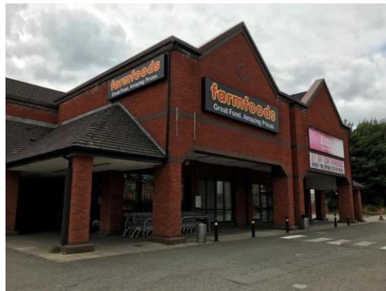
Figure 17 - View of the superstore
