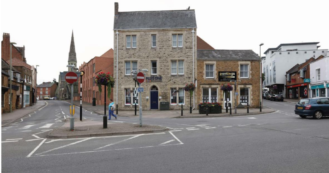
Figure 40 - View along Marlborough Road, showing built form providing an enhanced sense of enclosure in this location whilst retaining the Methodist Chapel tower as a key feature.
