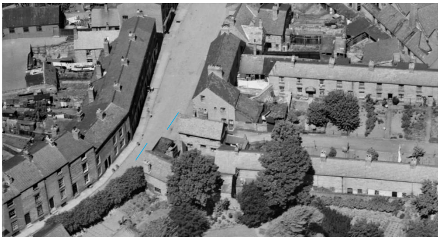
Figure 32: Note the buildings highlighted in blue and the range of terraces to the rear of both. No. 25 also has a domestic garden bound by hedges.
