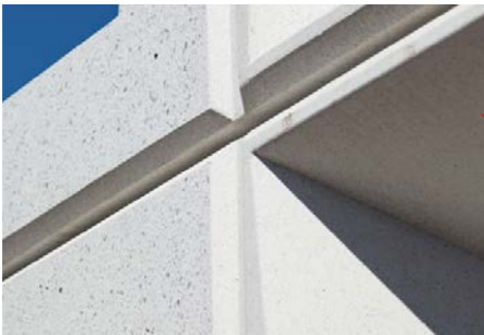
Slab Edge: pre-cast white concrete - acid etched
