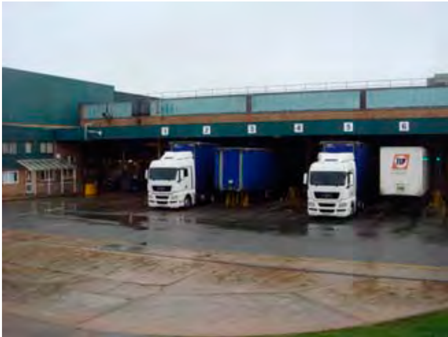
Plate 5: View of loading bay on south side of warehouse
