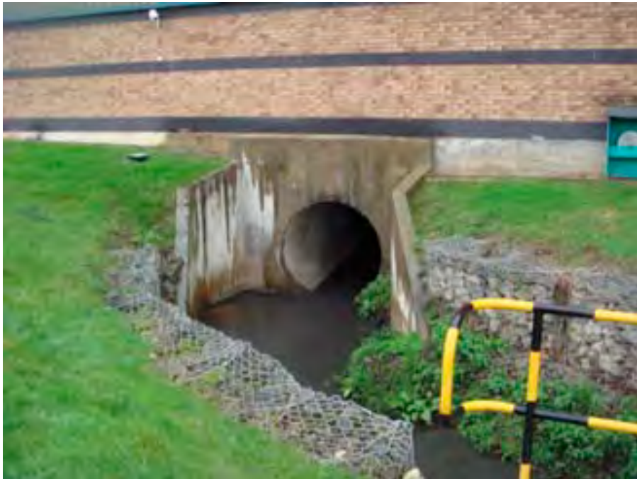
Plate 1: View of Birds Brook discharge from culvert beneath warehouse building.
