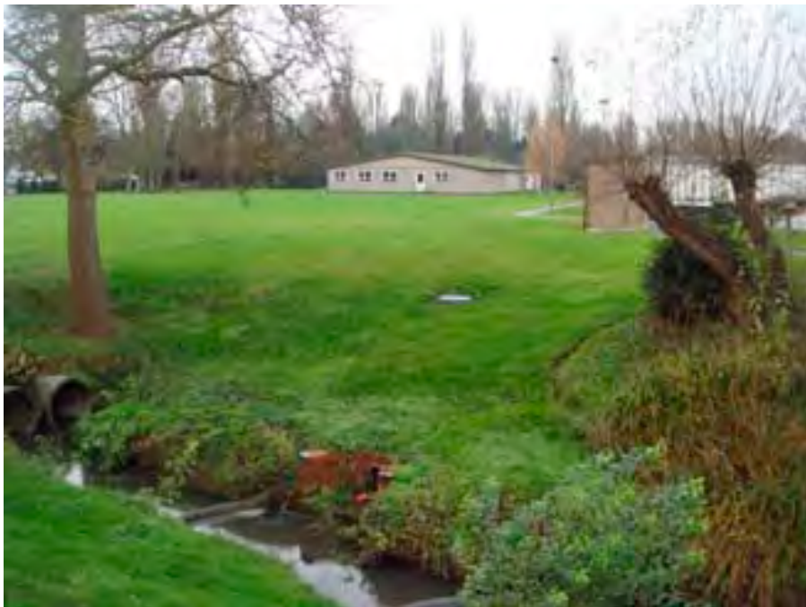
Plate 2: View across eastern site area towards vacant office building.
