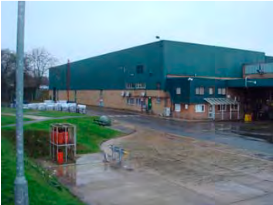
Plate 4: View of south west corner of warehouse unit. Location of former fuel filling station is in foreground on concrete apron.
