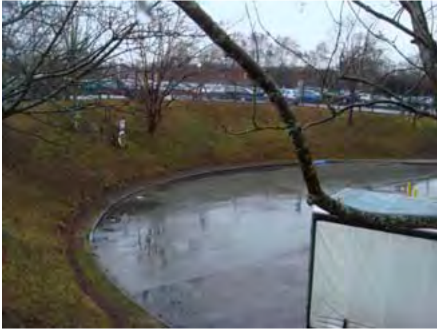
Plate 7: View of embankment on south west site boundary with Kraft car park beyond.
