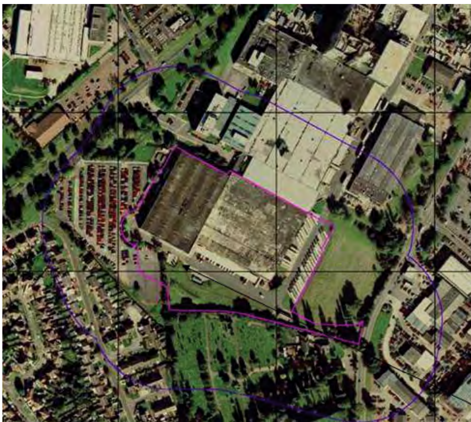
Location of Tanks
