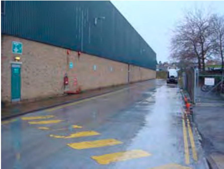
Plate 8: View of western flank of warehouse and access route.
