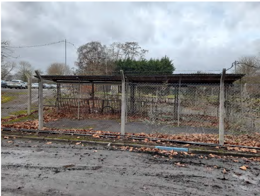
Photograph 14 – Disused bike storage area – possible asbestos containing materials.
