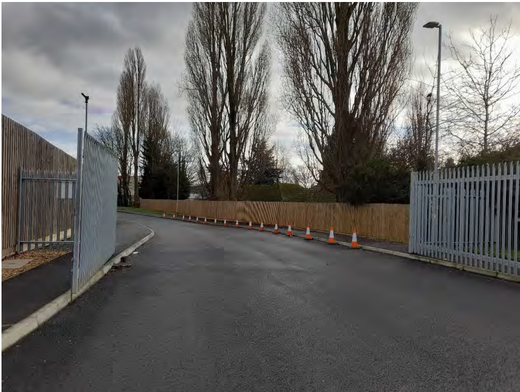
Photograph 1 – Access road to warehouse off Southam Road.
