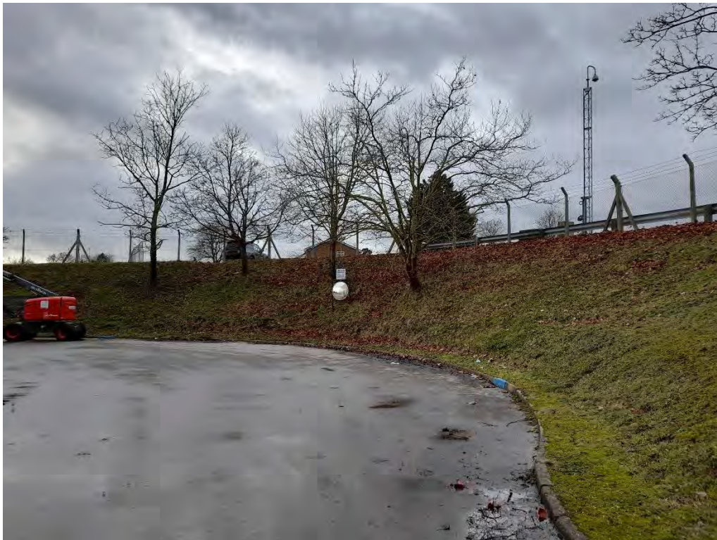
Photograph 18- Embankment (approx. 3 m high) between warehouse and car parking area.
