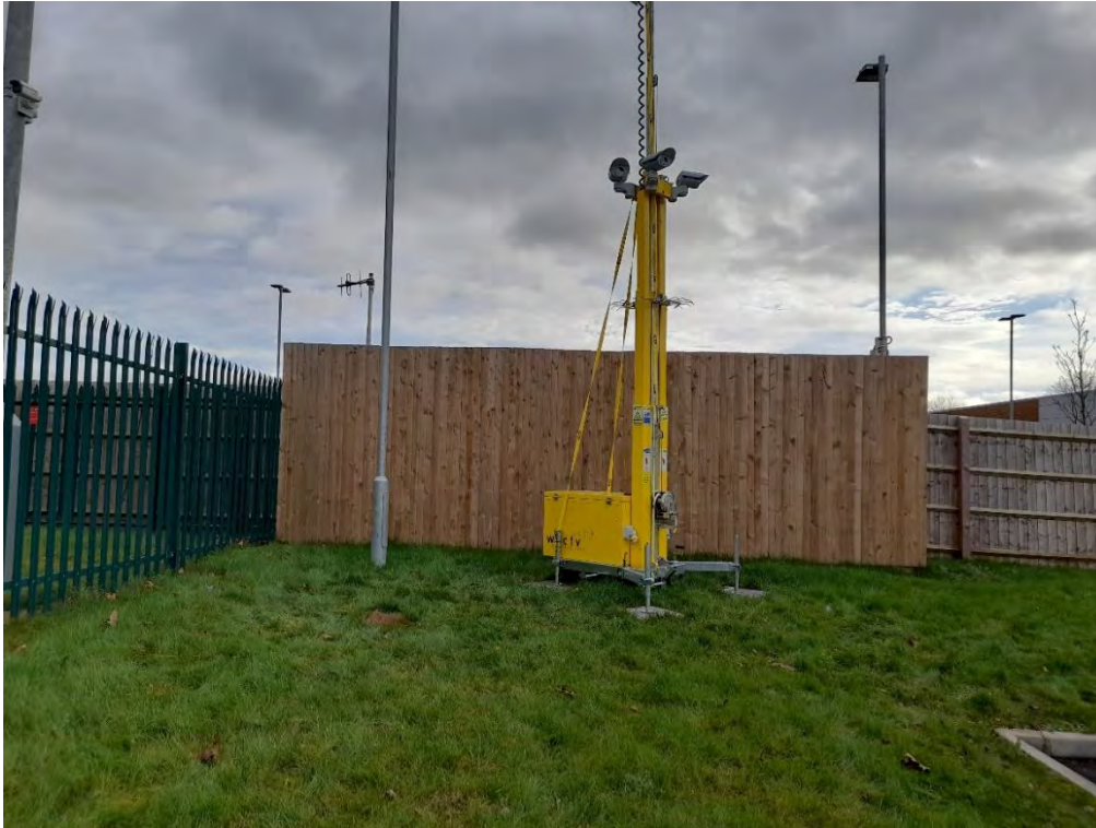
Photograph 7 – Substation with wooden enclosure in the north-eastern corner of the warehouse area (outside of Site boundary).
