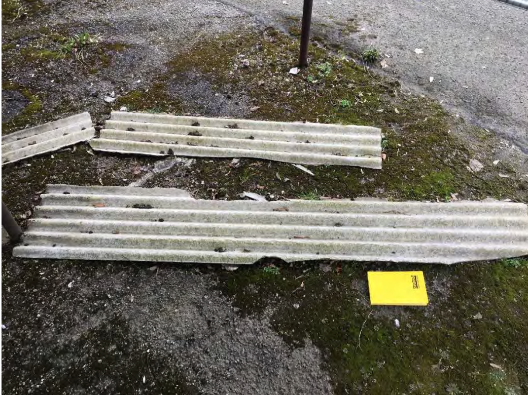
Photograph 45 – Fragments of suspected corrugated sheets containing asbestos.
