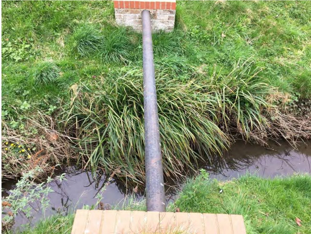
Photograph 39 – Pipe above the stream.
