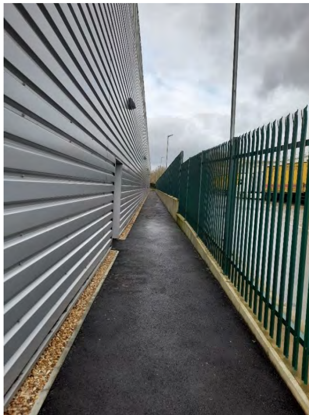
Photograph 8 – Pedestrian access walkway along northern elevation of warehouse.
