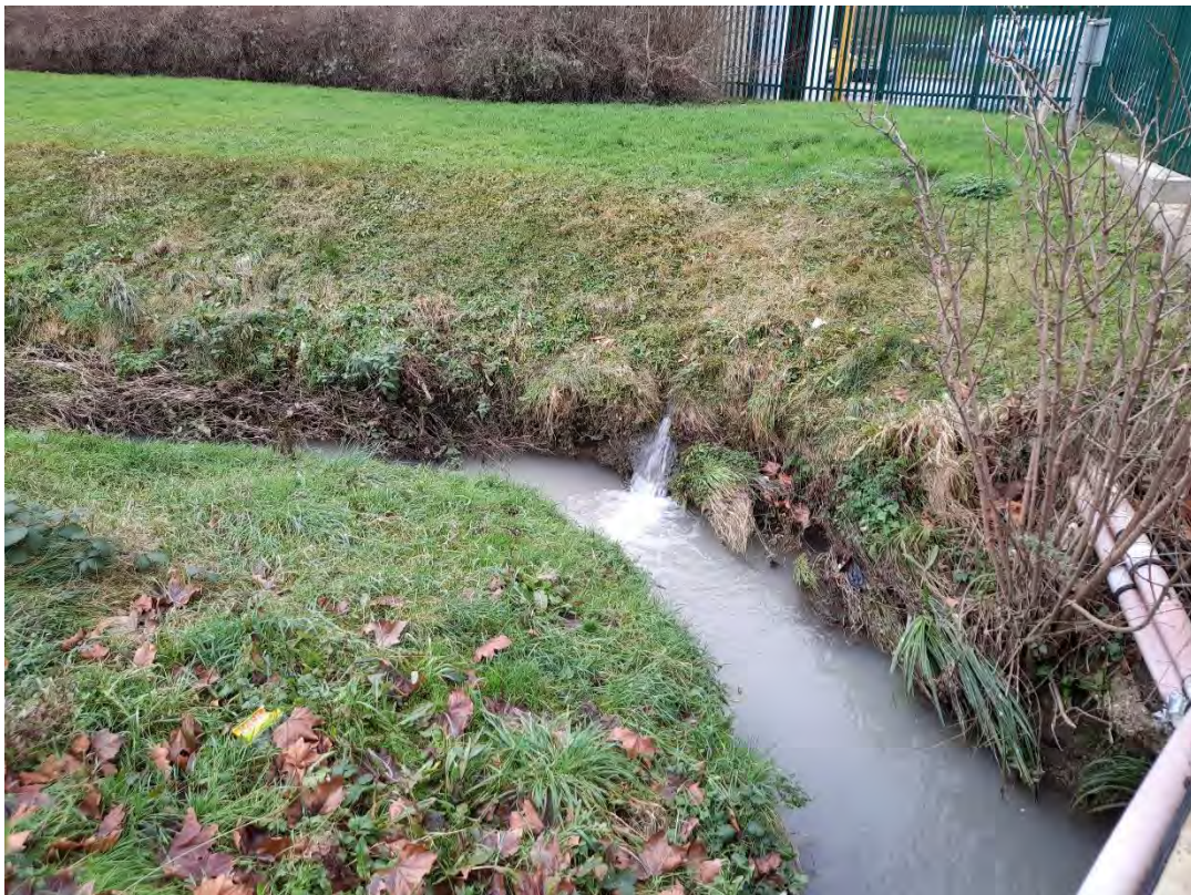
Photograph 12 – Discharge point into Bird Brook.
