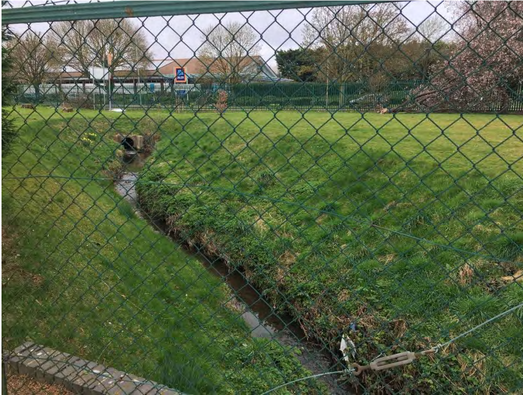
Photograph 37 – Culverted stream behind mesh fencing.
