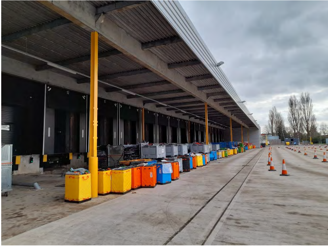
Photograph 5 – Southern elevation of warehouse with HGV loading bays.
