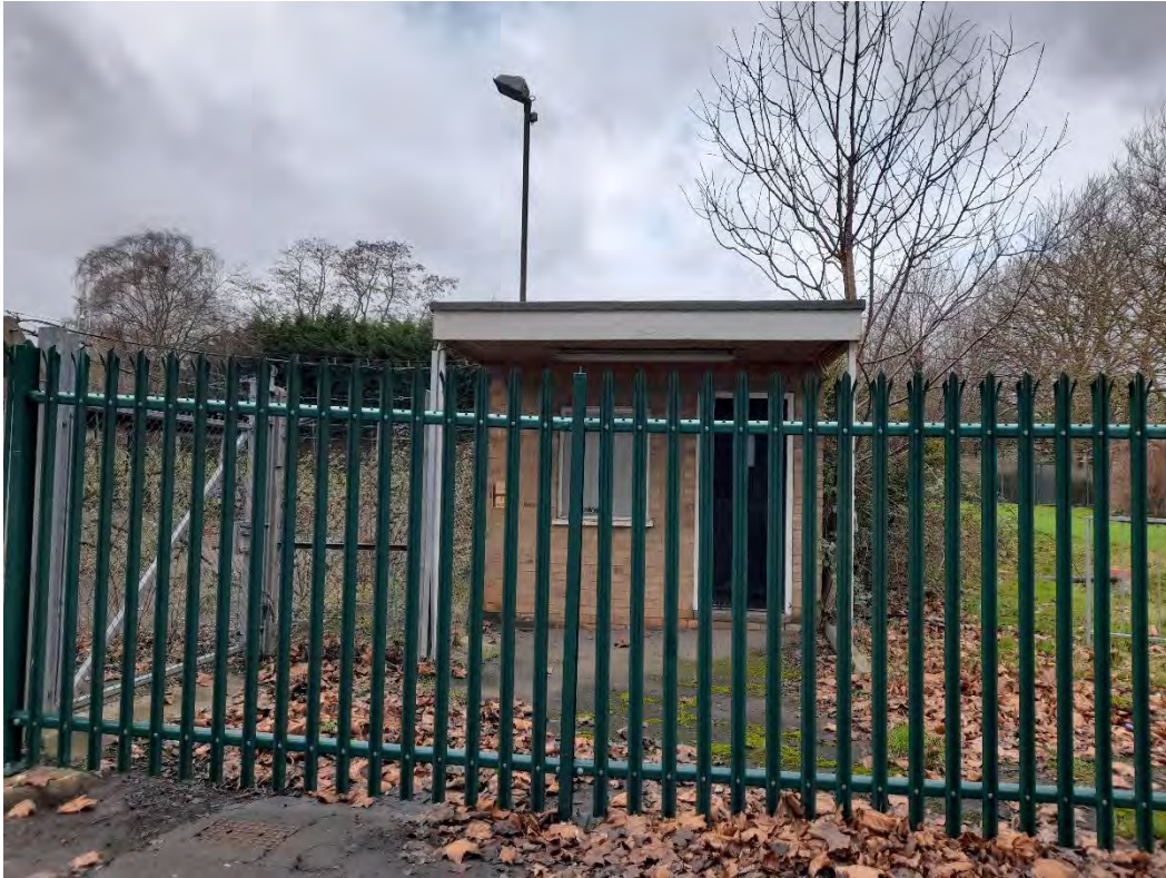
Photograph 13 – Maintenance building within car park area.
