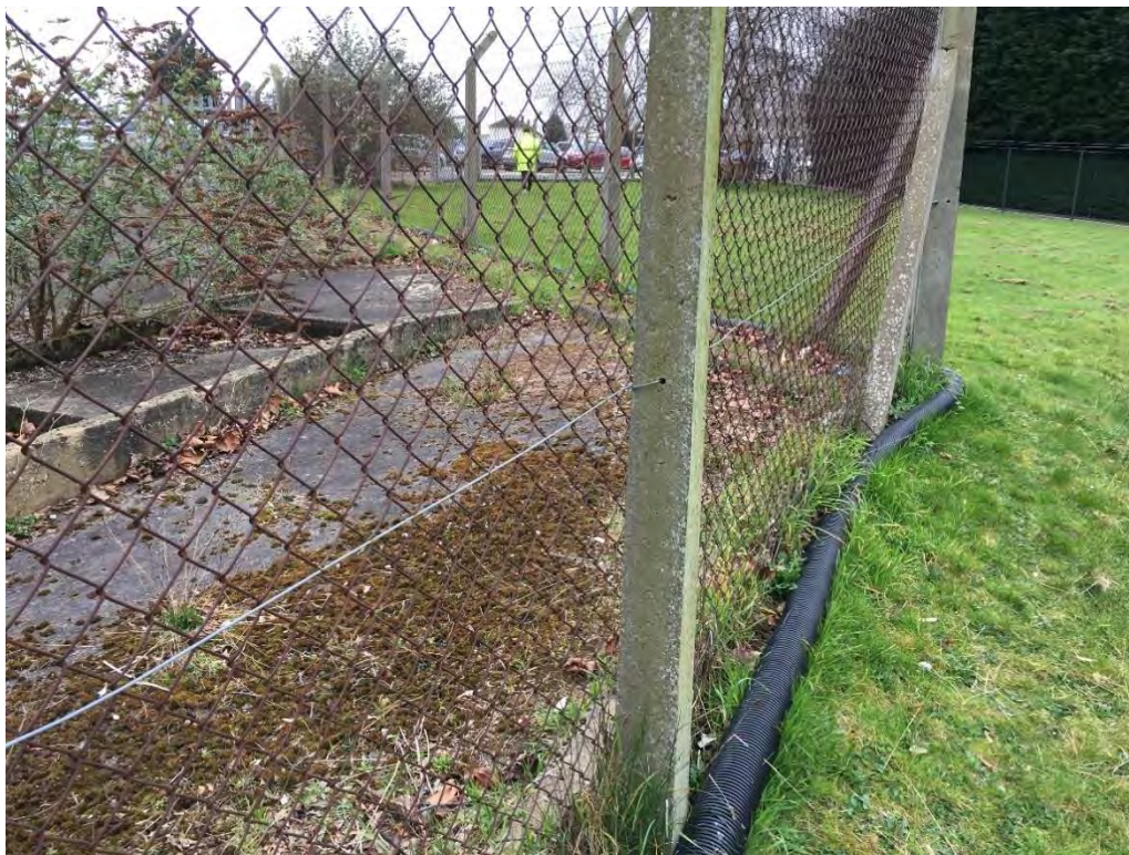
Photograph 42 – Above-ground (presumably) electric cables running to the maintenance building.
