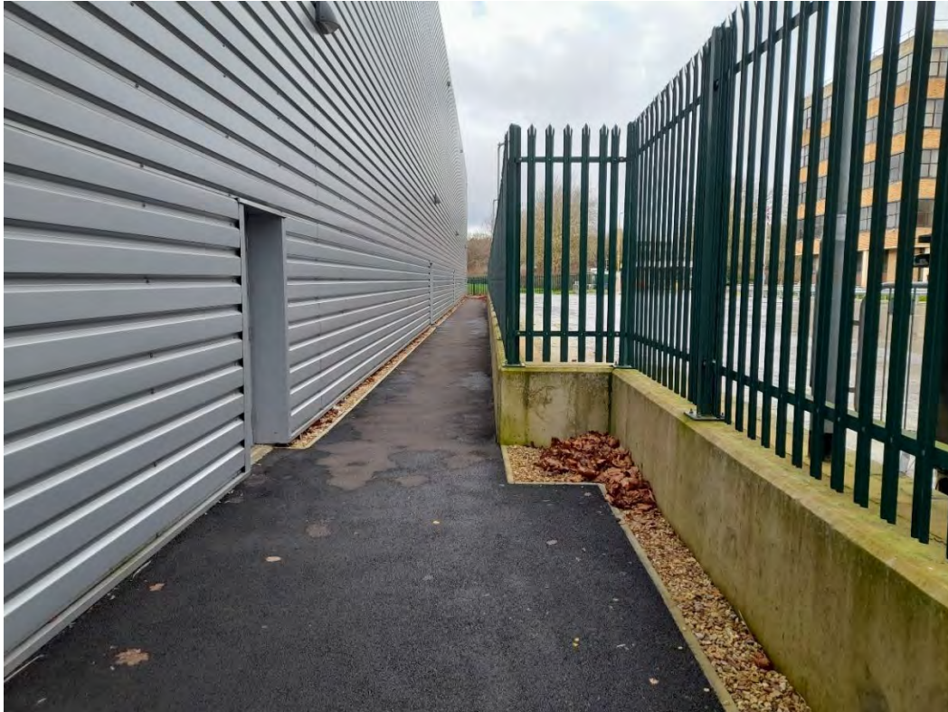
Photograph 9 – Levels of the adjacent plot (in the right of the photo) approximately 0.5 m higher than the subject Site. Looking north-west along the northern warehouse boundary.
