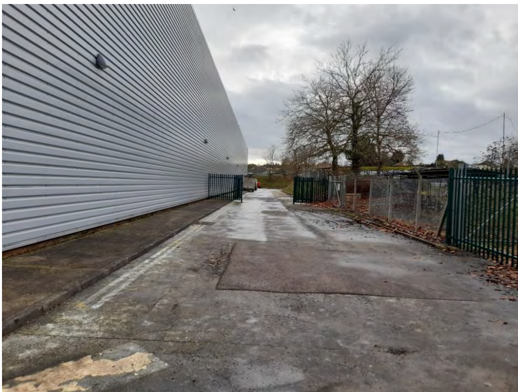
Photograph 10 – Concrete access road between warehouse and car park.
