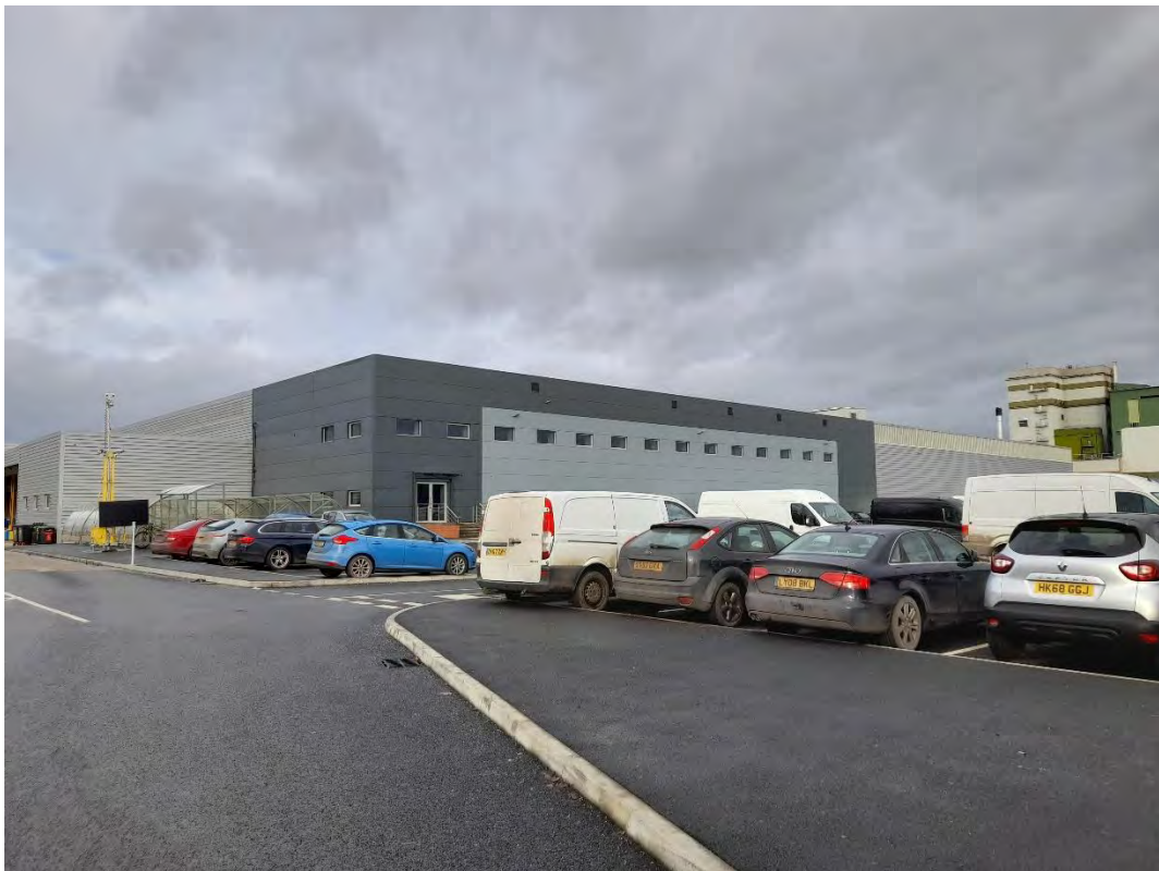
Photograph 4 – Warehouse building looking north.
