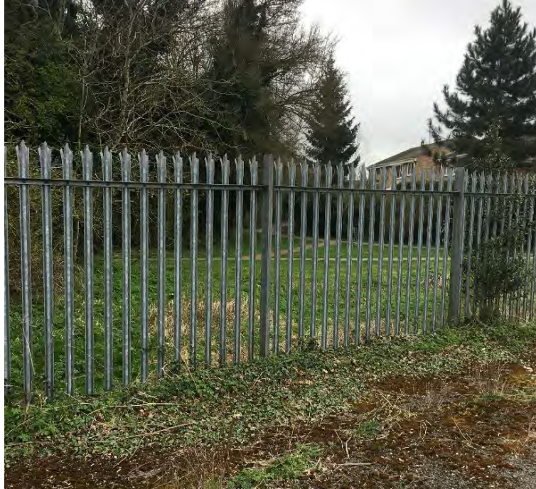
Photograph 29 – Metal fencing along the southern and western boundary.
