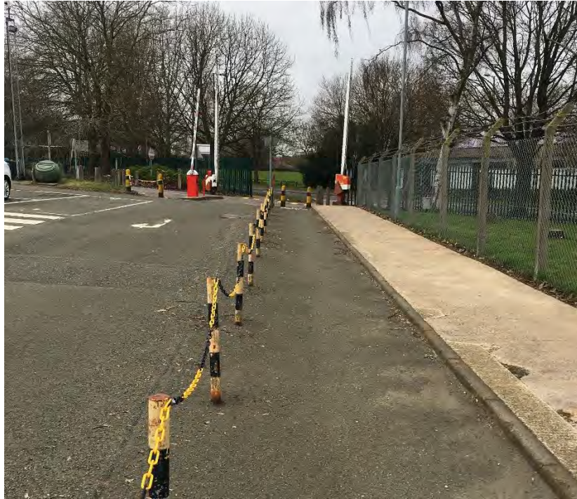
Photograph 35 – Pedestrian walkway along the car park adjacent to entrance.
