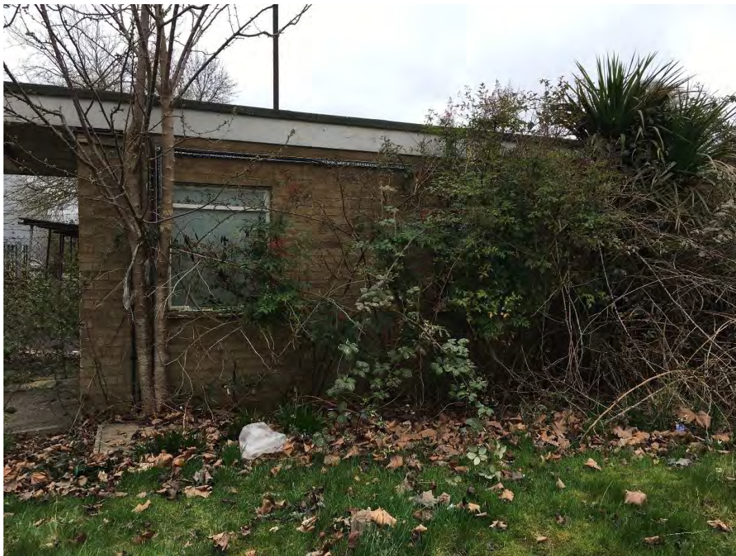
Photograph 40 – A small maintenance building in the north-east.
