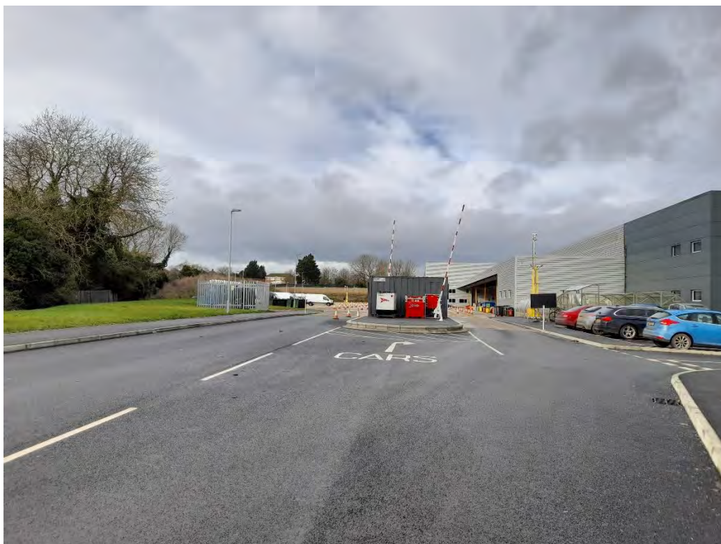
Photograph 2 – Warehouse extents looking north-west.
