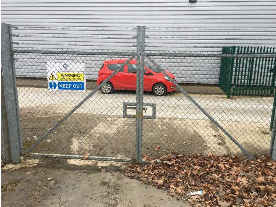
Photograph 27 – Metal access gate between car park and warehouse.
