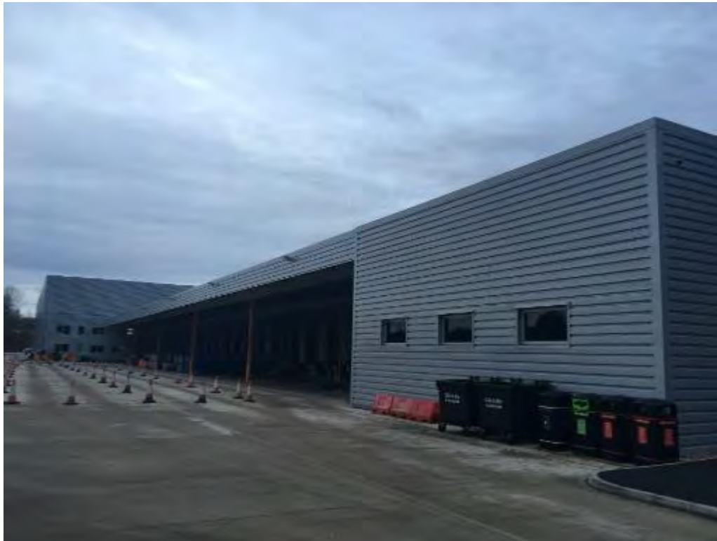
Photograph 11 – Large industrial warehouse
