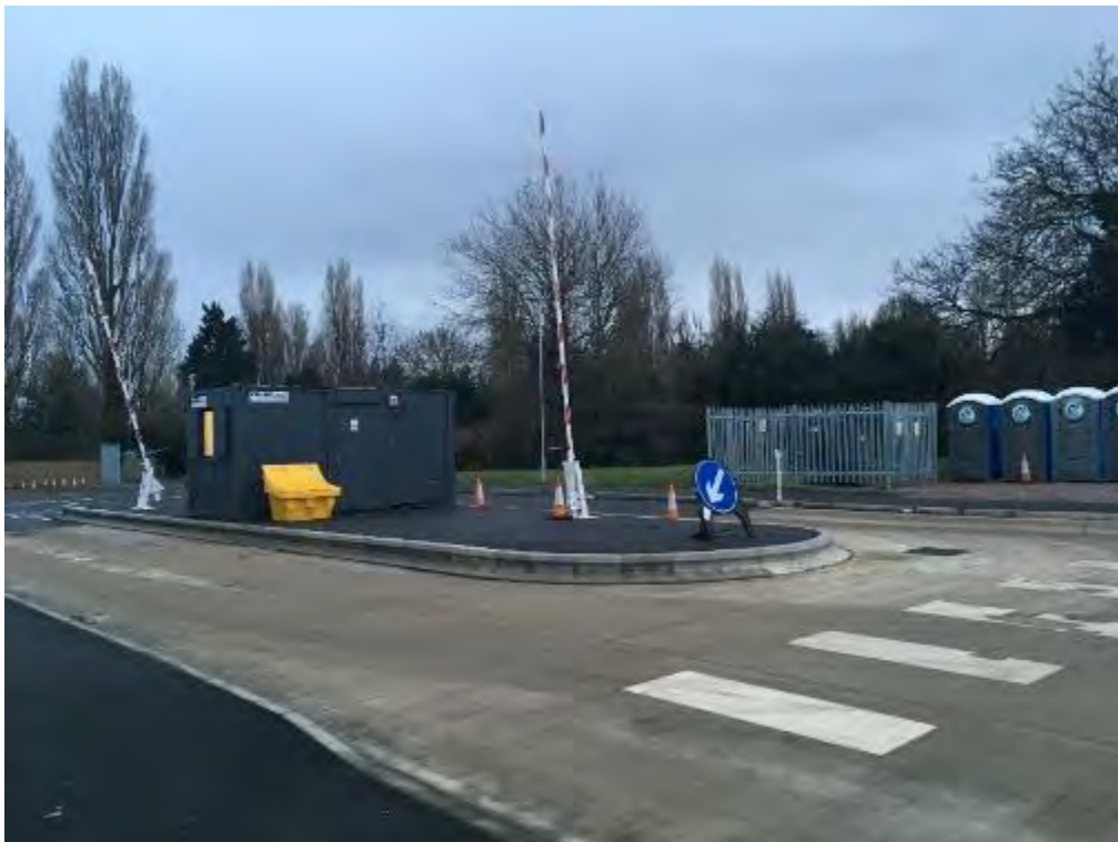
Photograph 12 – Security hut in the south-east of the Site
