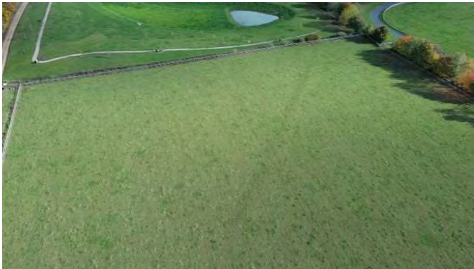
Aerial view of the site, towards the eastern field boundary. Shows the drainage lagoon beyond the timber fence boundary.
