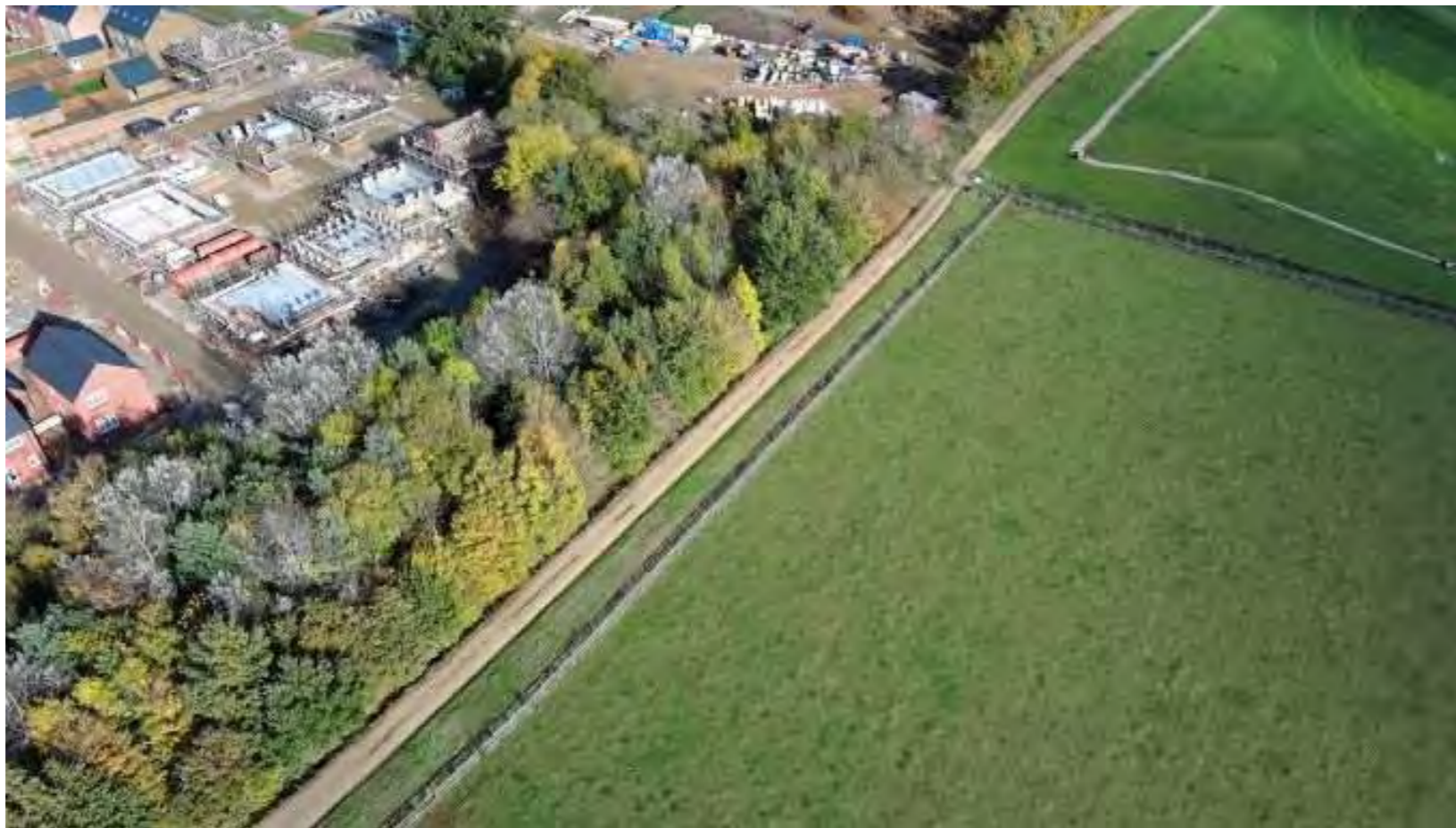
Aerial view of the site, towards the north eastern corner of the site. Shows the track, woodland and the adjacent development.
