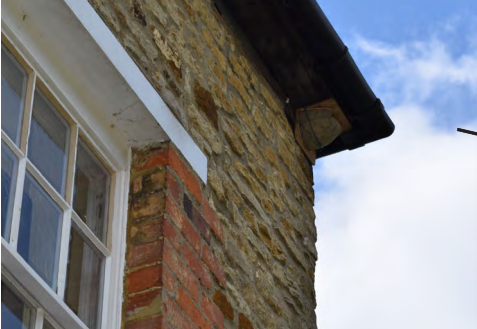
Swift Box on north elevation
