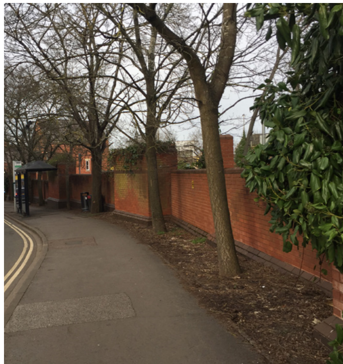
Existing Retaining Wall to Calthorpe Street
