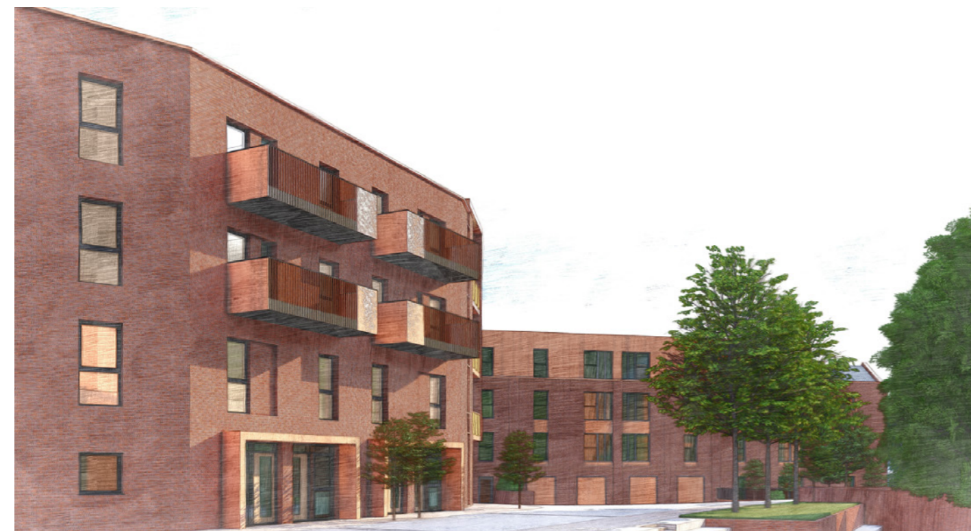
Balconies to Block E overlooking the Church Square Play Plaza
