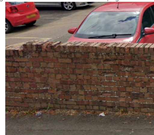
Indicative proposal for new red brick boundary wall, with garden wall bond and bullnose brick coping
