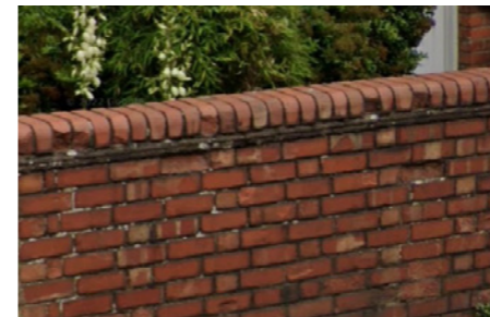
Bull nose brick coping to Marlborough Road
