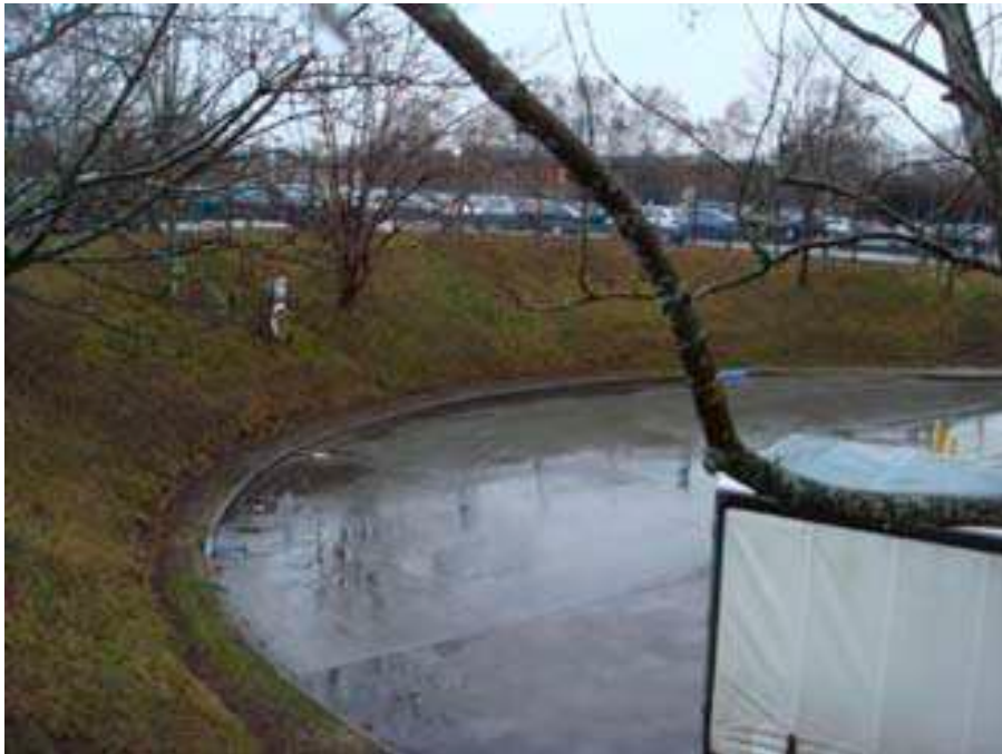
Plate 7: View of embankment on south west site boundary with Kraft car park beyond.
