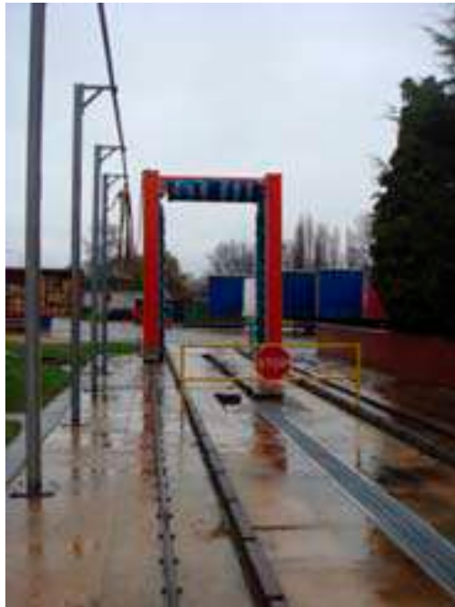
Plate 3: View of truck wash with truck park and trailer park behind.
