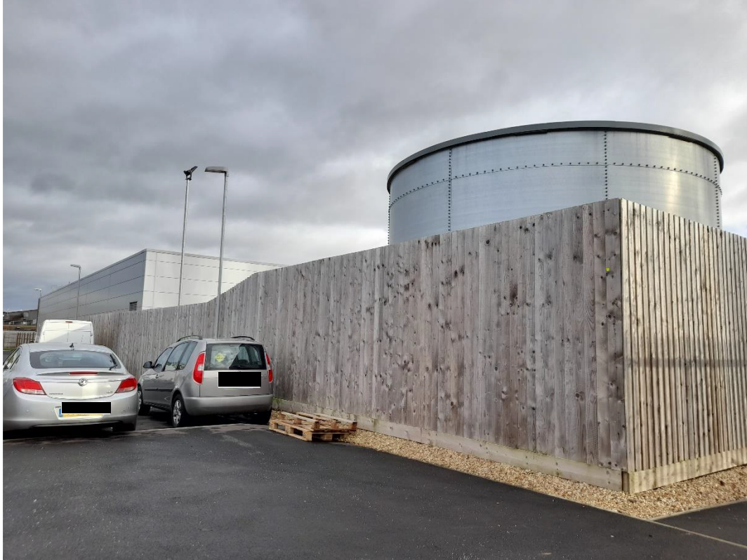
Photograph 25 – Off-Site water tank associated with the neighbouring Waitrose store.
