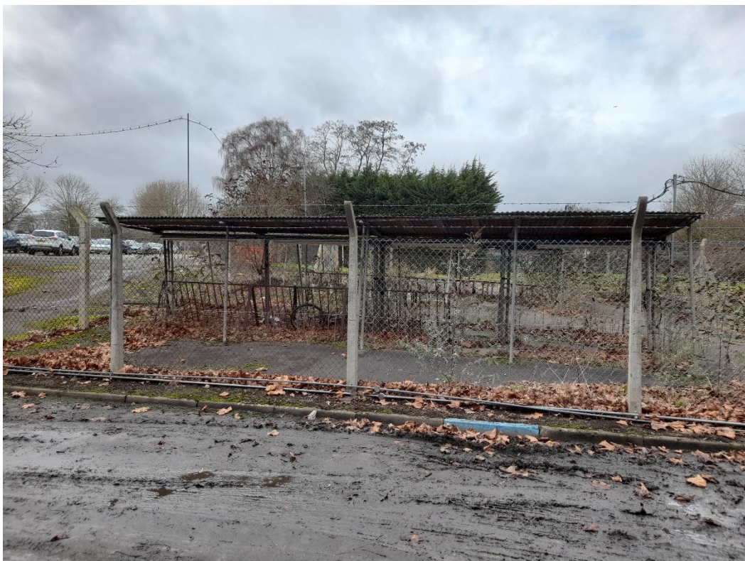
Photograph 14 – Off-Site disused bike storage area adjacent to western Site boundary
