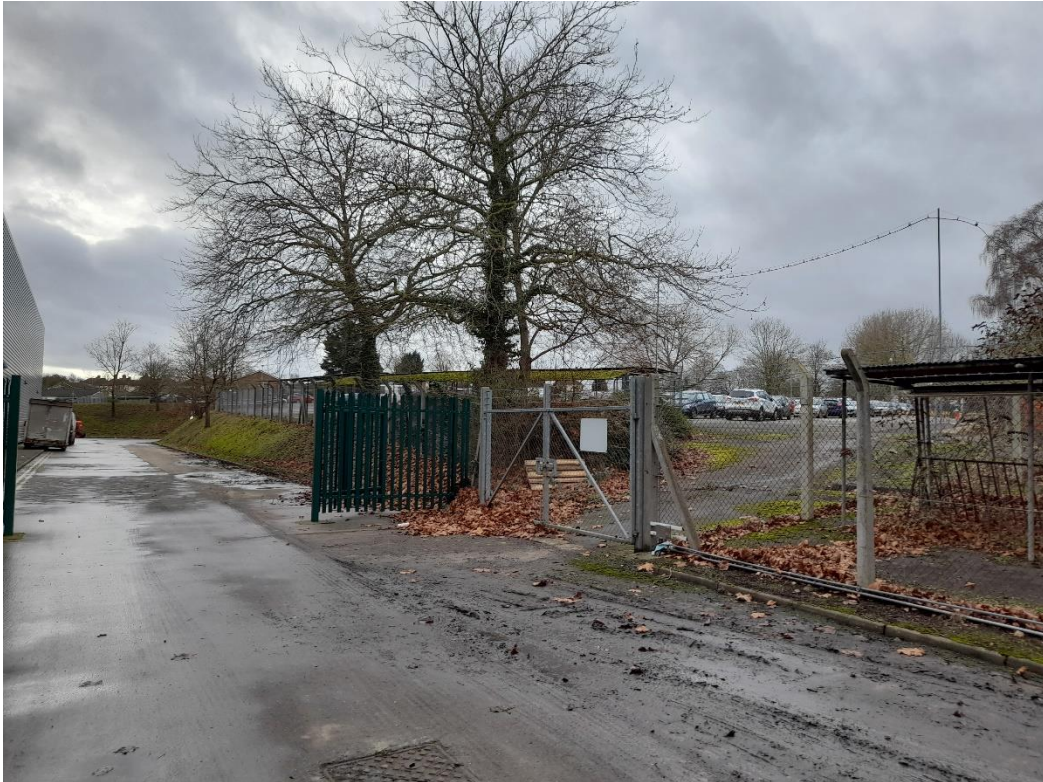
Photograph 15 – Access point leading into adjacent car parking area along western Site boundary.
