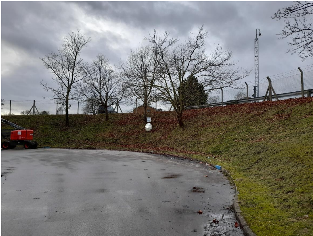
Photograph 18- Embankment (approx. 3 m high) along western and southern Site boundary
