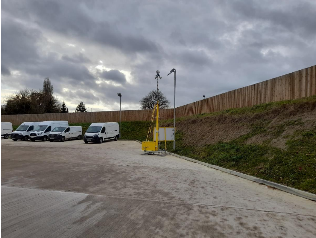
Photograph 19- Wooden fencing atop the embankment in the south
