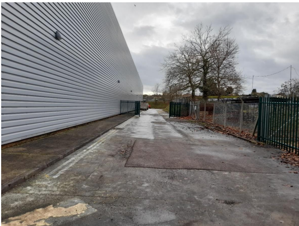
Photograph 10 – Concrete access road along western Site boundary
