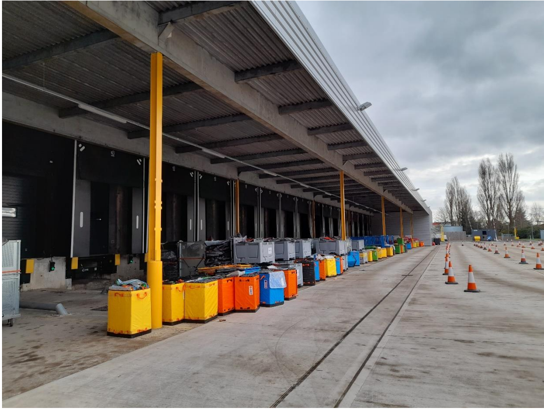
Photograph 5 – Southern elevation of building with HGV loading bays
