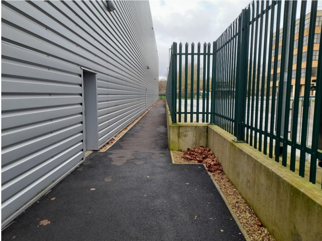
Photograph 9 – Levels of the adjacent plot (in the right of the photo) approximately 0.5 m higher than the subject Site. Looking north-west along the northern Site boundary
