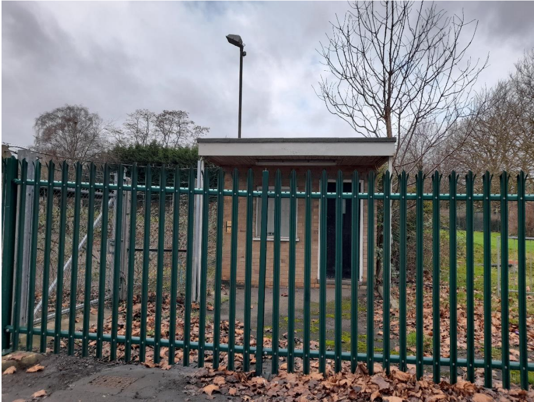
Photograph 13 – Off-Site structure adjacent to western Site boundary (unknown use)
