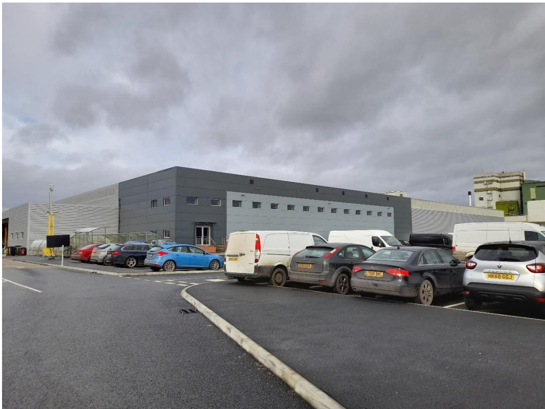
Photograph 4 – Warehouse building looking north
