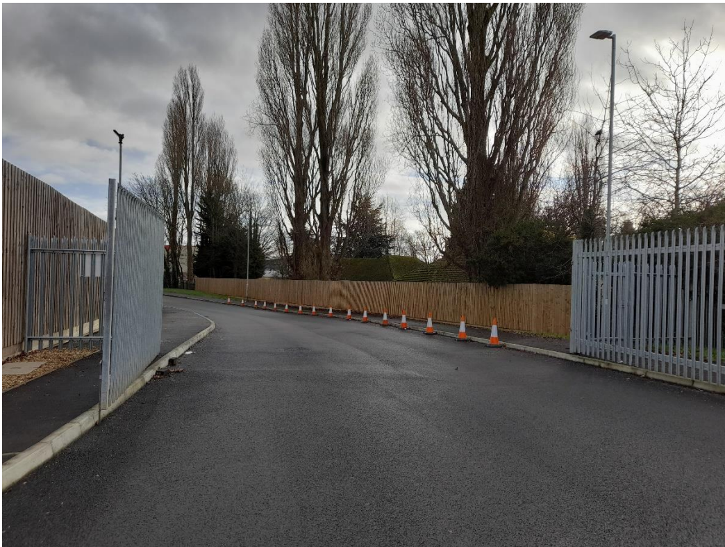
Photograph 1 – Access road in the south-eastern corner off Southam Road
