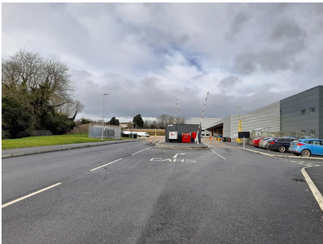
Photograph 2 – Site extents looking north-west
