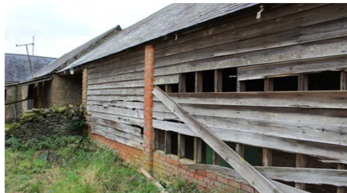
Fig. 15 - Brick and timber alterations
