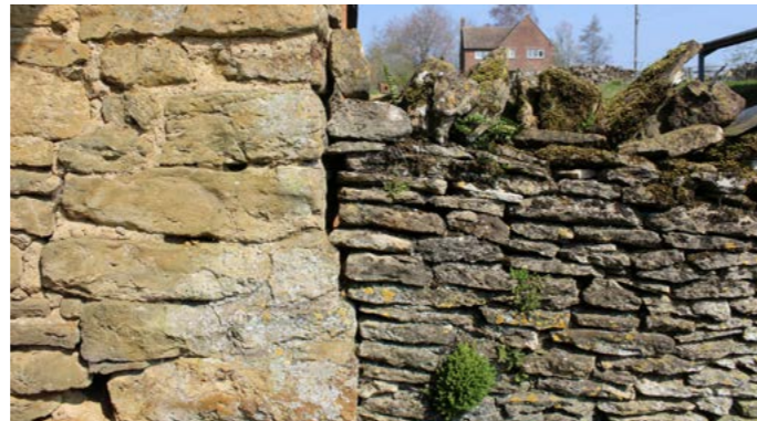
Fig. 14 - Coursed ironstone rubble and walling stone
