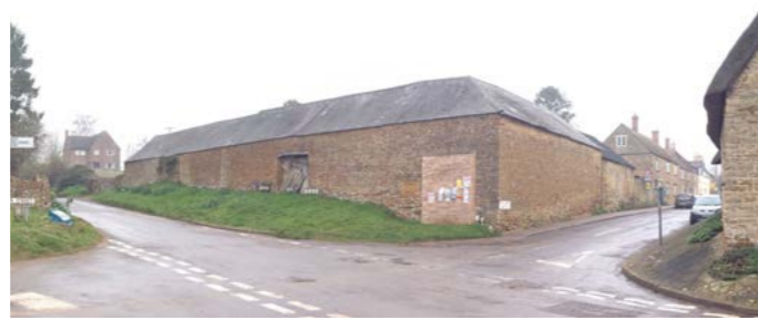
Fig. 13 - External appearance from the crossroads
