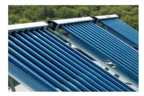
Figure 11: Solar thermal hot water panels.
