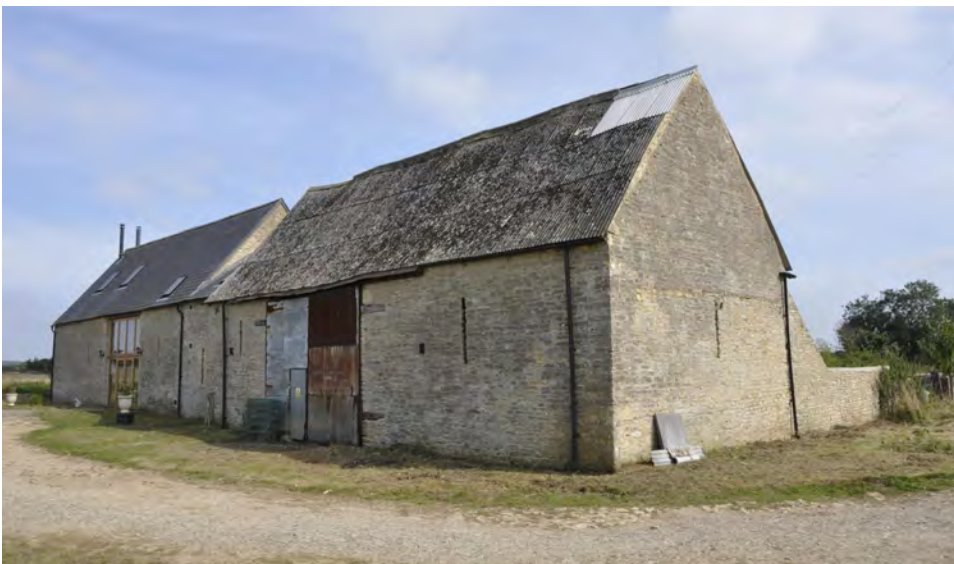
The two barns from the south looking north
