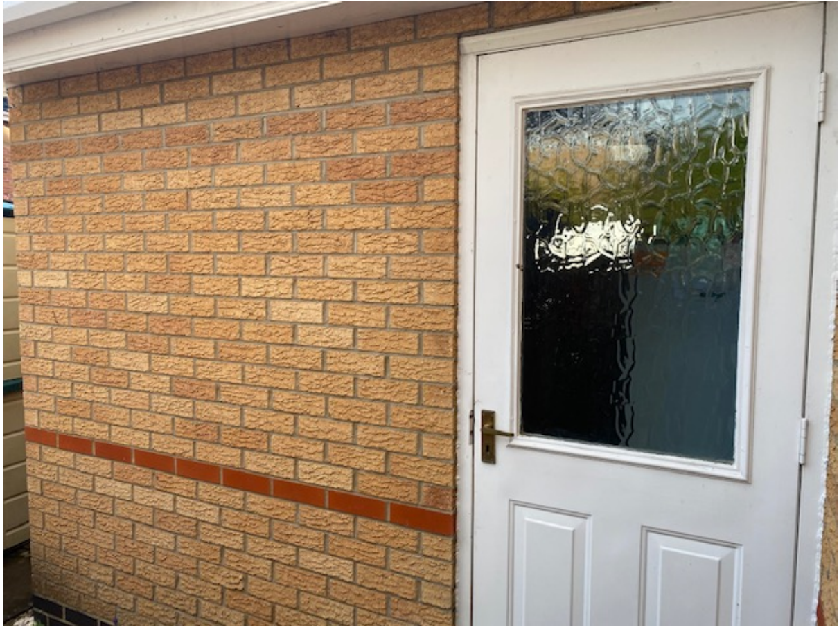
Rear elevation of garage
