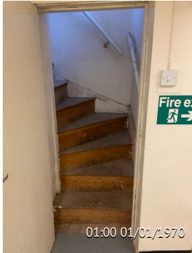
first floor 15, stairs up to second
