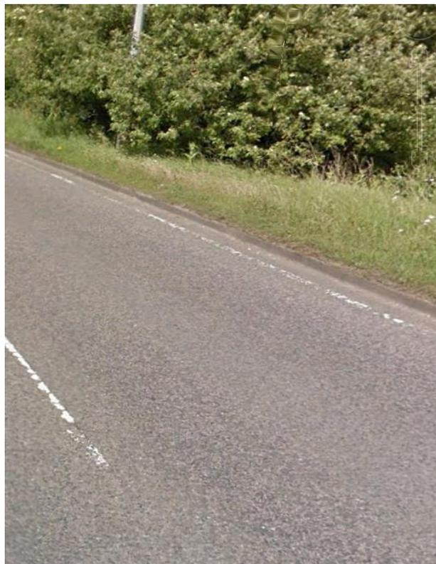
**Figure 14 Overall Indicator of Pavement Risk “Sound” Condition**
