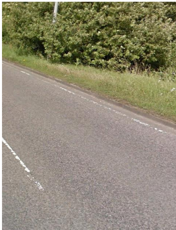
Figure 14 Overall Indicator of Pavement Risk “Sound” Condition
