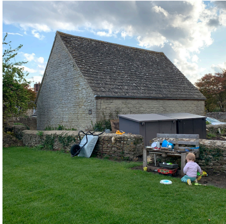
Fig. 2 - Oubuilding on neighbouring land
