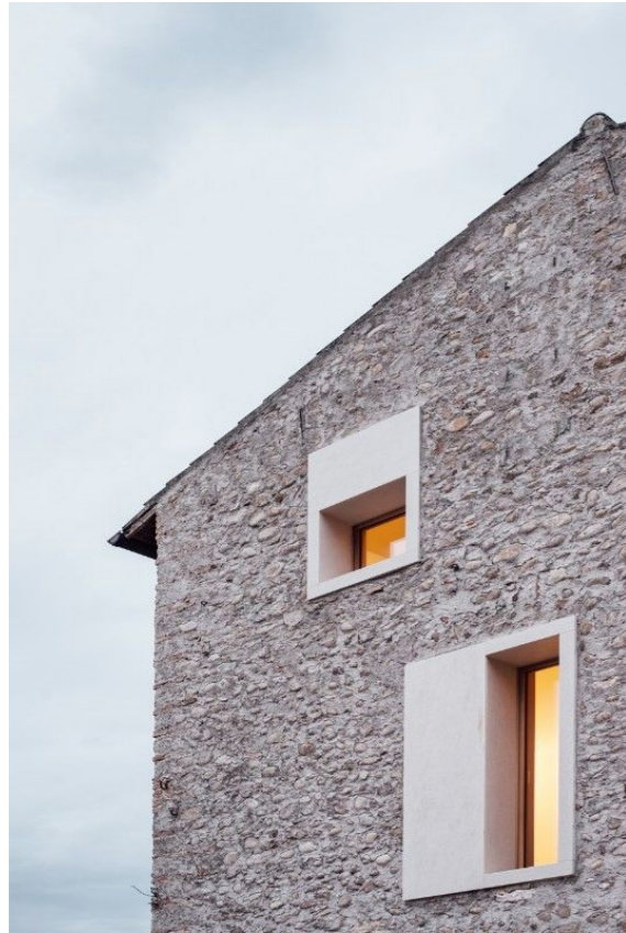
Fig 7. Using natural stone with worked stone to introduce contemporary detailing
