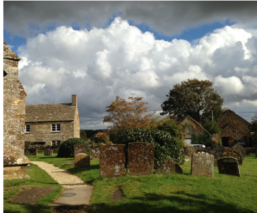
Fig. 3 - Chancel Cottage from the Church - the proposed outbuilding will not be visible from this view as will sit behind the existing outbuilding of the neighbouring land
