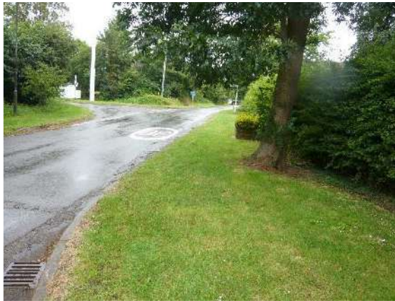
Insufficient vertical clearance beneath existing tree canopy
